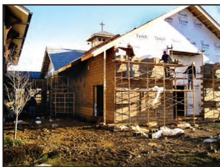
Brick is added to the exterior.
