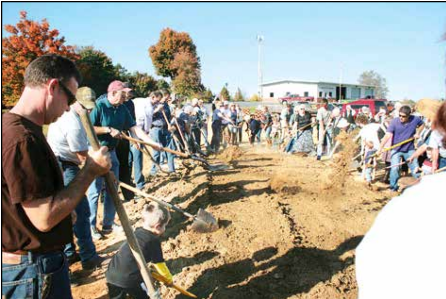
Groundbreaking. Photo by Danny Thompson
