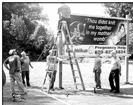
The photo of the billboard construction at St Lawrence Church is at top left.
