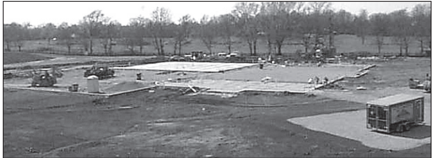
Holy Spirit Catholic Church (Spirit I - offices, catechetical space, parish hall & kitchen spaces) viewed on April 9, 2009, looking north with concrete slab on grade work in progress. Submitted Photo
